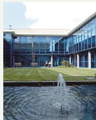
NHS Canford house clinic, Bournemouth, UK. VRF
